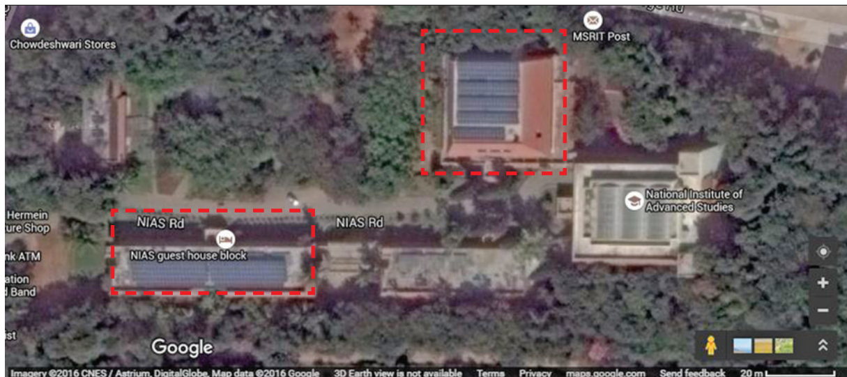
Figure 7 100kWp solar power plant at NIAS
